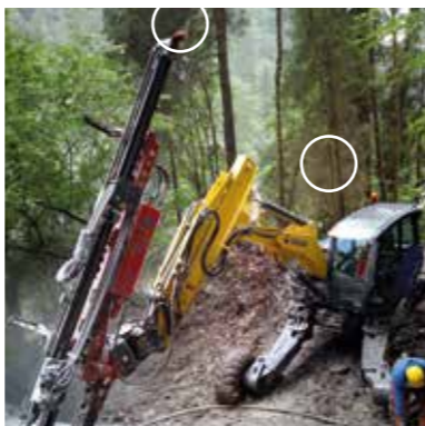
Example of the use of RS193rM* as a fixed point on different surfaces and for the exact alignment of the drill carriage.
