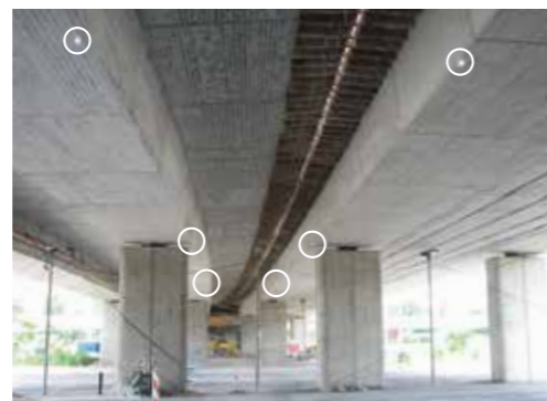
Observation of bridges
